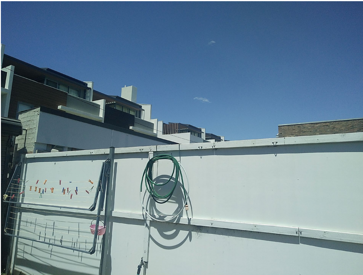
fence on southern boundary viewed from rear yard of site
